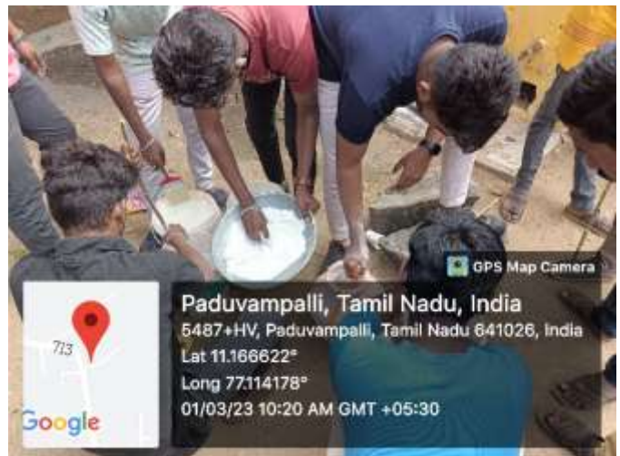
Preparation for School compound white wash
