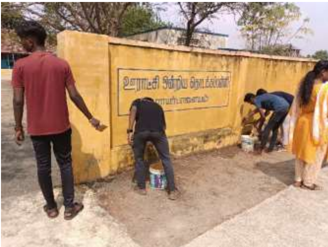
Painting work – school compound wall
