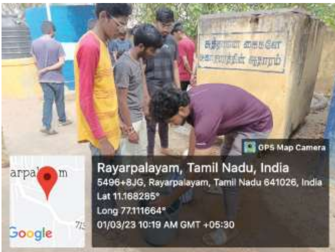
Preparation for School compound white wash
