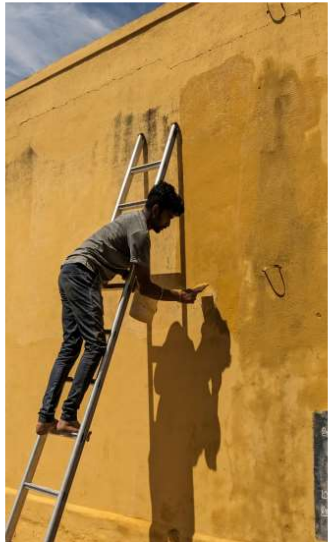
Painting work – school compound wall
